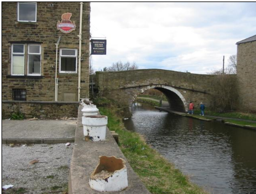
Canalside – Listed bridge
