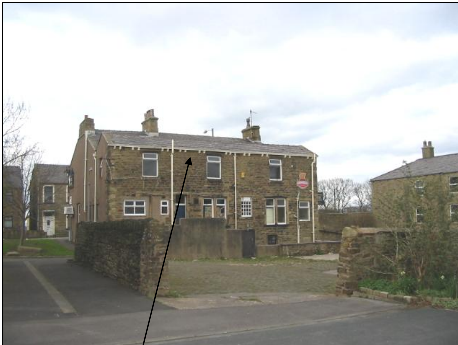
Rear of building; yard and access from Water Street
