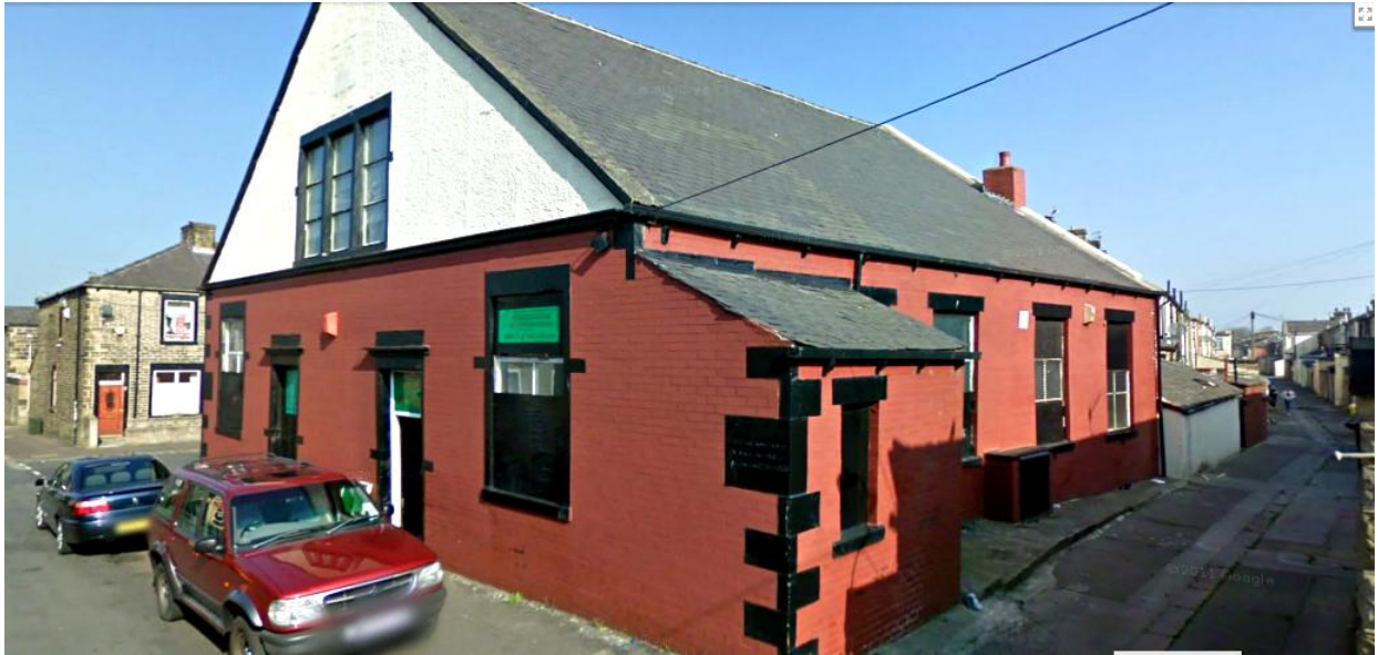
No.1 Bright Street frontage
