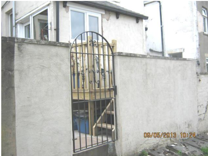
View of decking in rear yard
