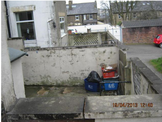
View towards rear yard at 4 Brunel Street
