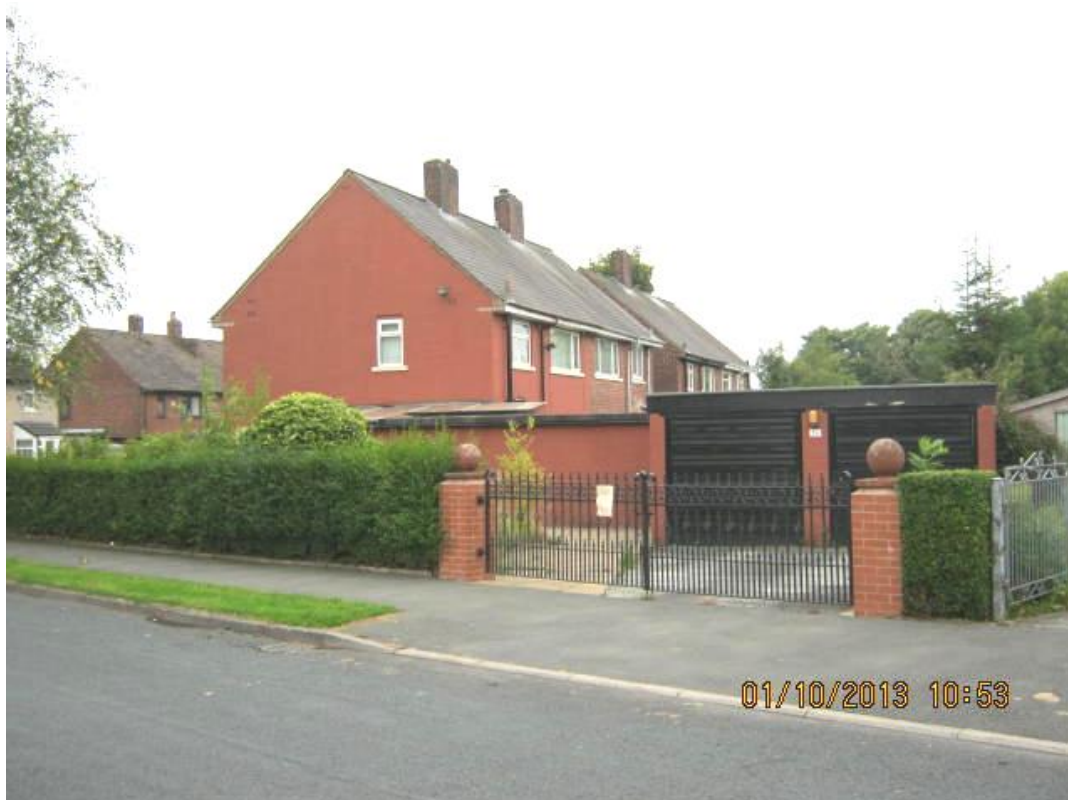
Side/rear of 28 Ennismore Street
