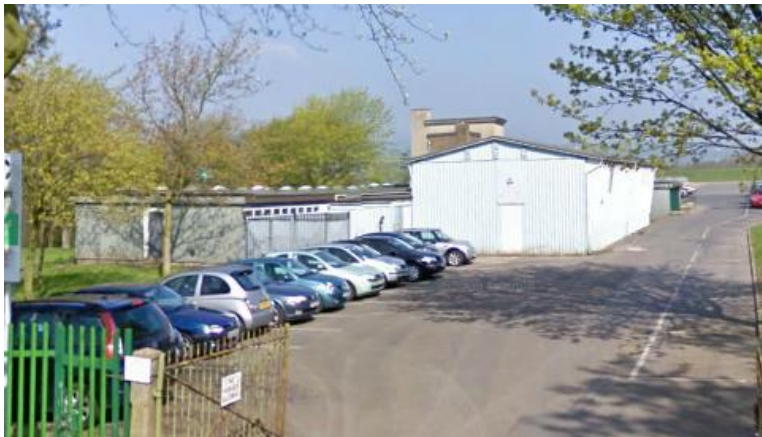
Existing building – view from Windermere Avenue
