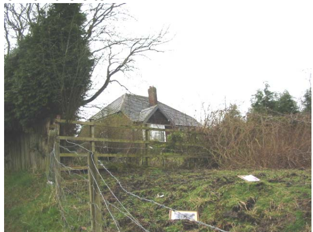
rear of existing bungalow
