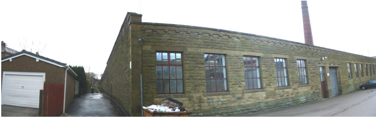
back street rear of Harrison Street
