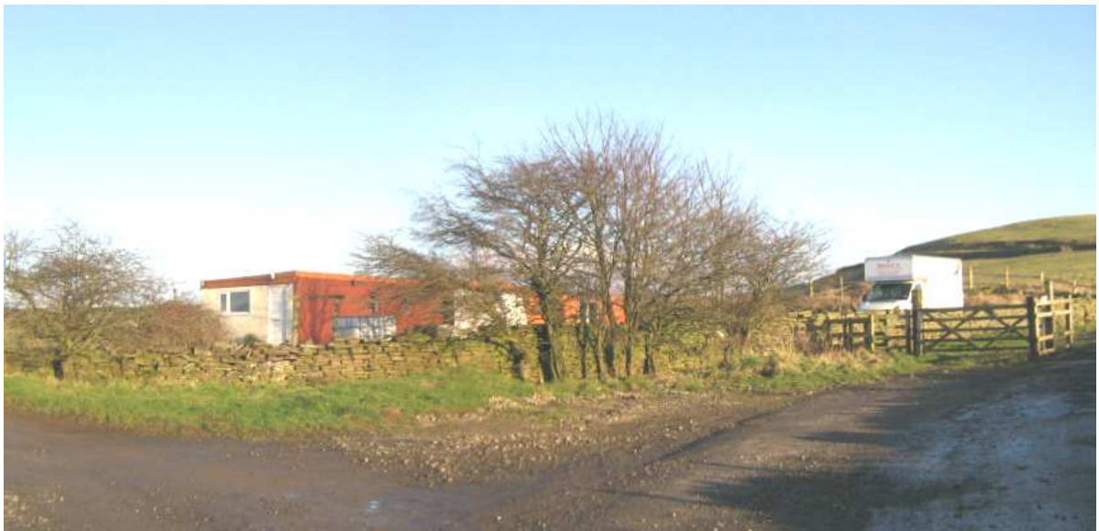
Converted kennel building viewed from lane
